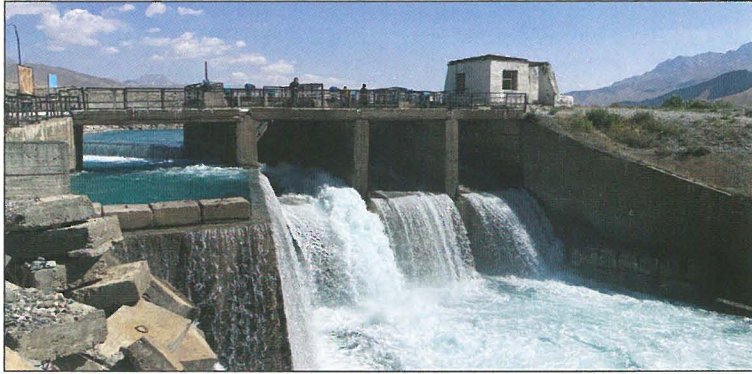
The existing weir at At-Bashi, Kyrgyzstan.
