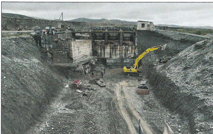
Construction works at the At-Bashy plant. Below: Start of earthworks in September 2024. Below right: Advance by the end of November 2024.
